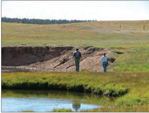
Photo 14. Severe Bank Erosion
