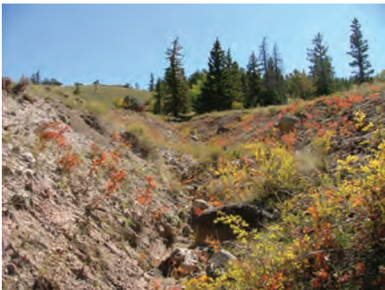
Photo 9. Eroded Gully on Western Portion of Knoll
